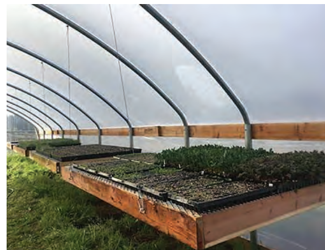
A view of the newly build greenhouse.
